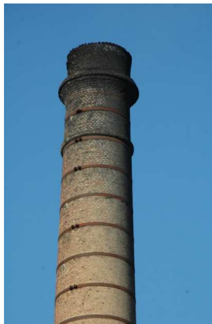
Figure 6: Detail of a chimney illustrates the craftsmanship of brickwork, using bands of metal strips to provide added strength and rigidity against the wind
